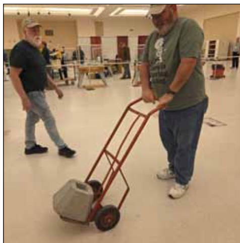
Heavy cement blocks secure the booths' poles. Steve Talmadge lifts them into place.
