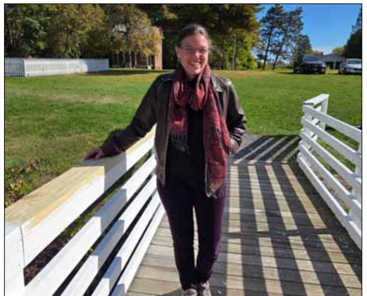
Johanna Batman inspects and approves our work
