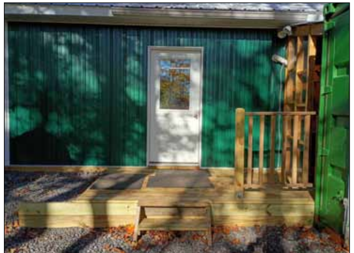
New deck at the shop provided by Mike Guiliano and Greg Lapp
