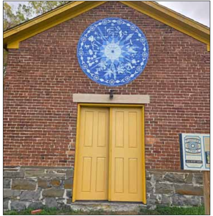
The new doors installed
