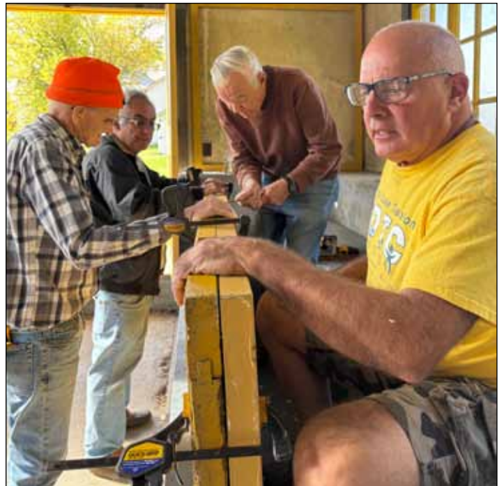
Lee aligns an old door with the new as Charlie mortises the new for hinge placement
