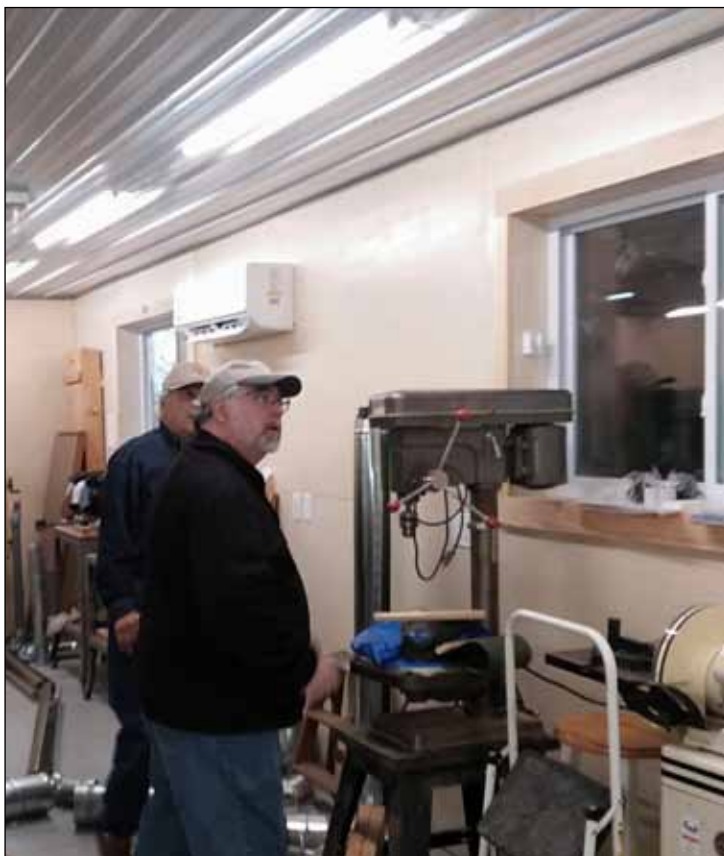
Andy Champ-Doran and Pat DiStefano lay out the piping system
