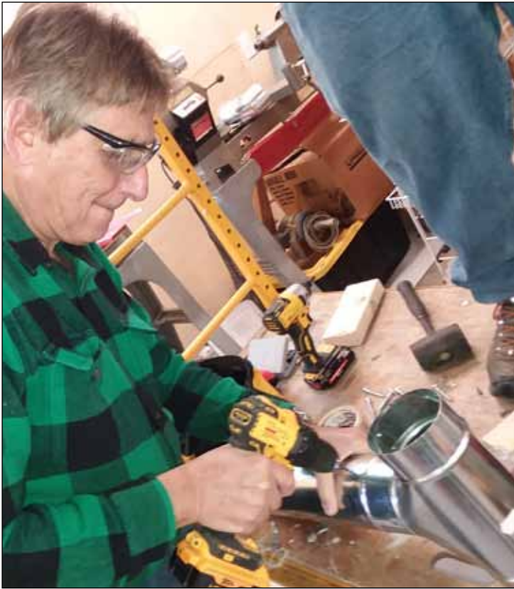
Steve Schoenberg attaches sections of the duct collection piping
