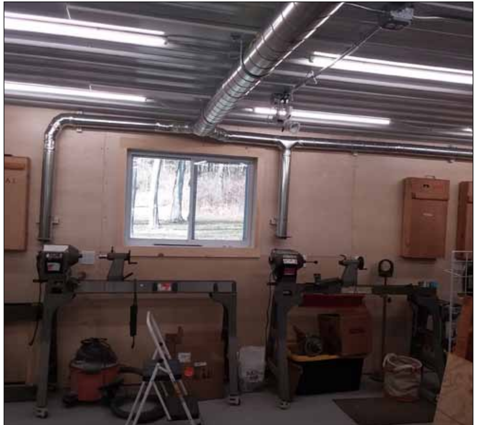
The finished wall with drops to the equipment placements
