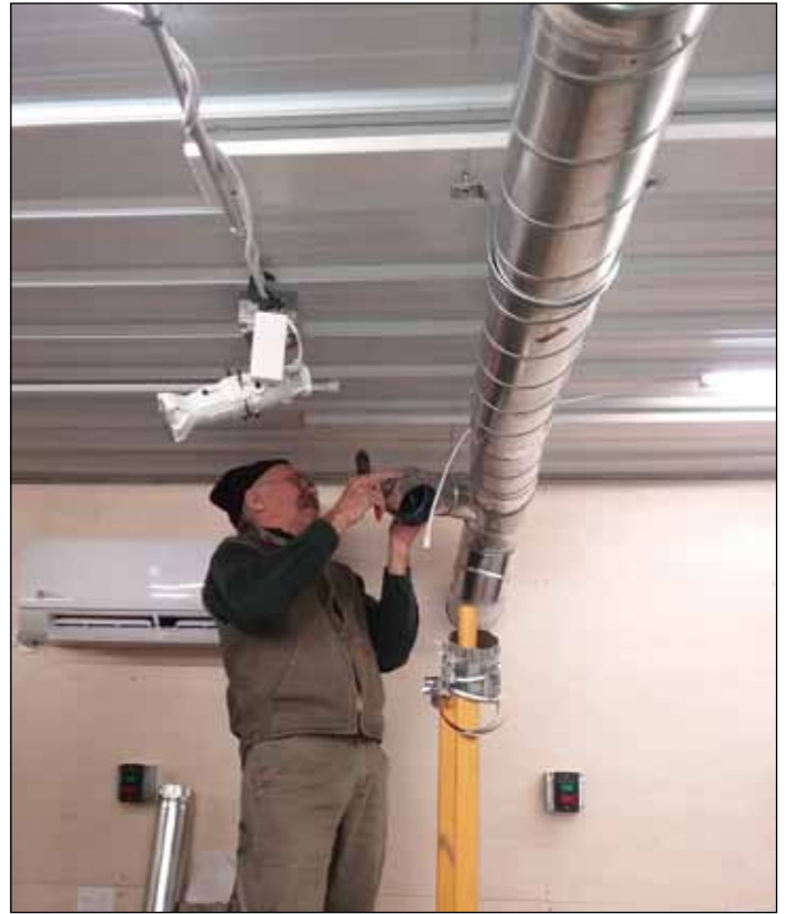
Ron Roberts secures the main pipe to the ceiling
