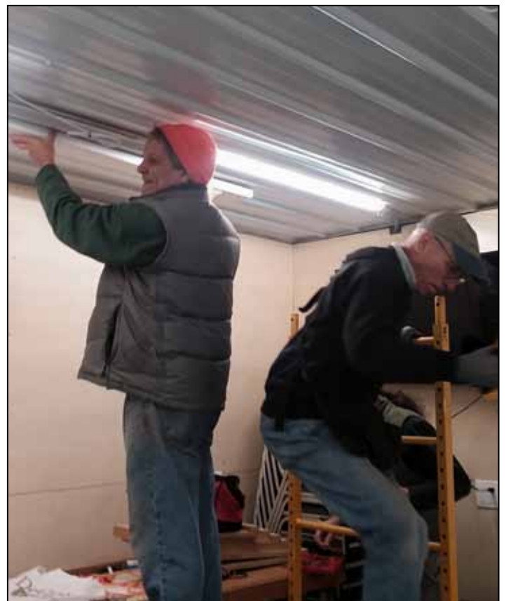
Mike Guiliano and Andy Moss install spacers on the metal ceiling to anchor the pipes
