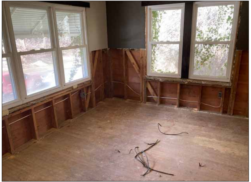
Walls cut away to 18 inch waterline
