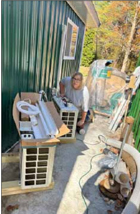
Kay McCampbell puts the final touches on the mini-split installation
