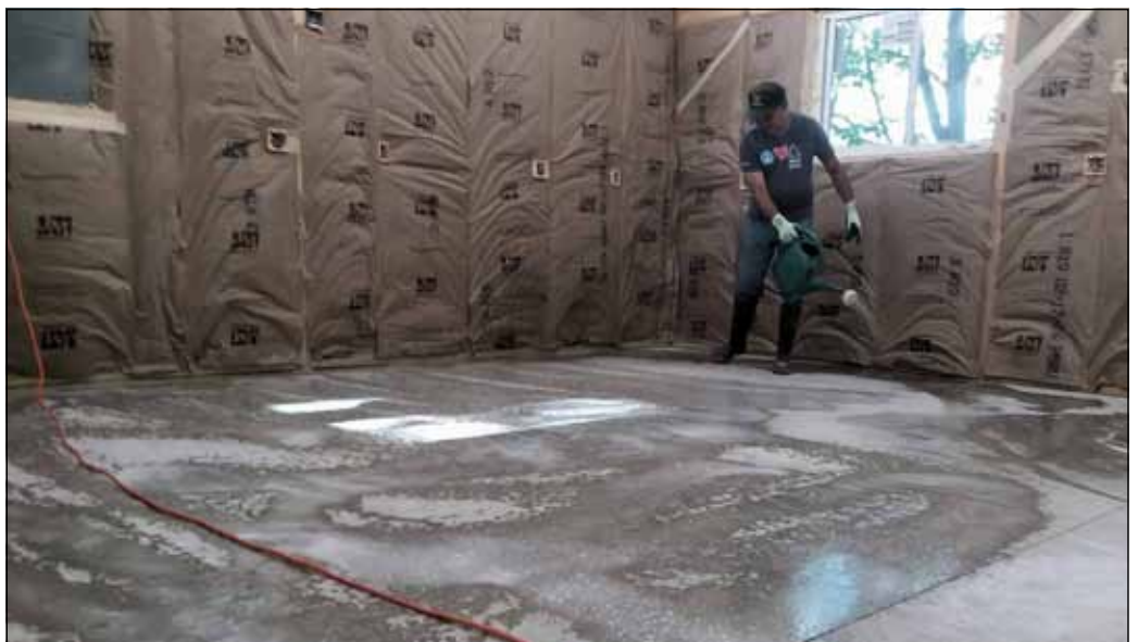
Mike Giuliano spreads the acid wash. It is then scrubbed into the concrete and rinsed off. It will take several days to dry.
