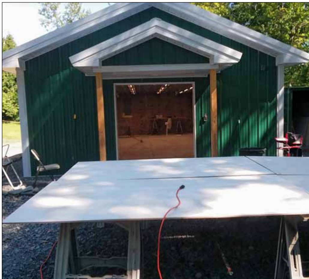
Maple plywood panels are sealed with several coats of polycrylic and set to dry.
