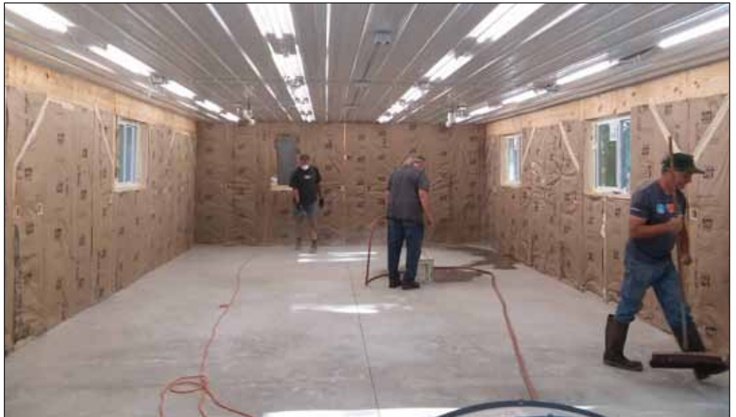
The shop floor is cleaned and ready for acid wash.
