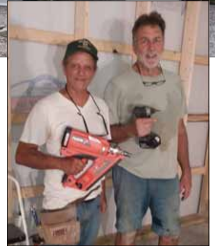
Mike Giuliano and Greg Lapp help with interior framing
