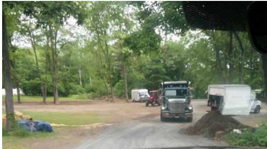
Many yards of fill dirt were trucked in to raise the site level
