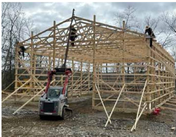
*An example of the builder's work in progress for another customer. The concrete slab is poured after the poles have been set.*
