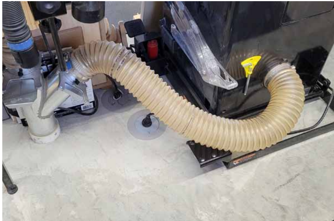
Paul's dust collection hoses under his radiant heat concrete floor
