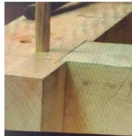
Pegs draw in the timber parts' joinery
