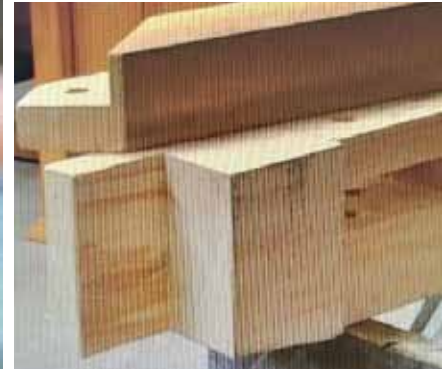
Brace reveals corresponding holes for beam
