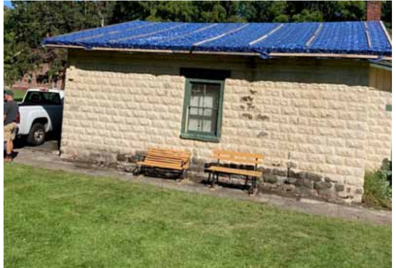
The roof is saved!
