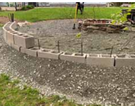
Concrete block as foundation
