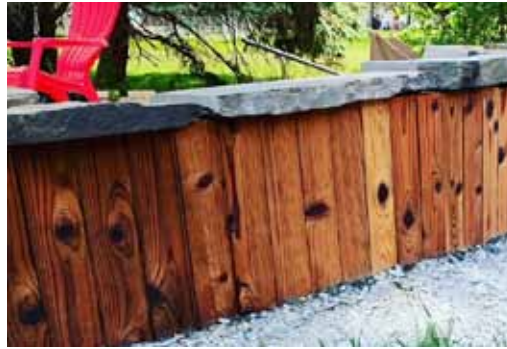
Redwood over the block makes an attractive wall.
