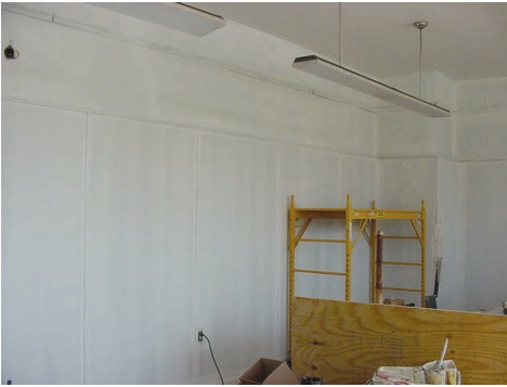
Prime coat of paint completed on the walls and trim.
