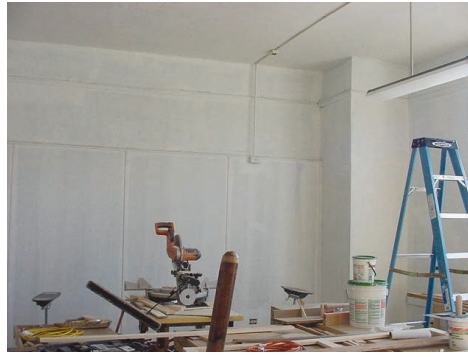
Prime coat of paint completed on the walls and trim.
