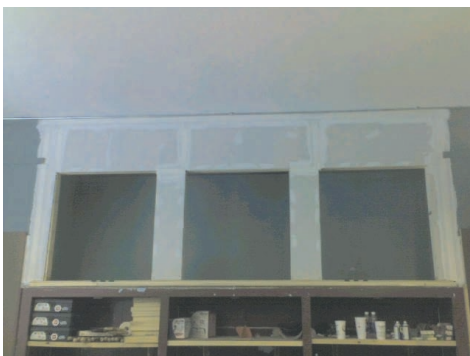
Sheetrock and taping completed on closets.
