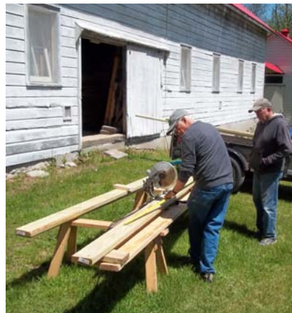
Deck's planks are cut on site
