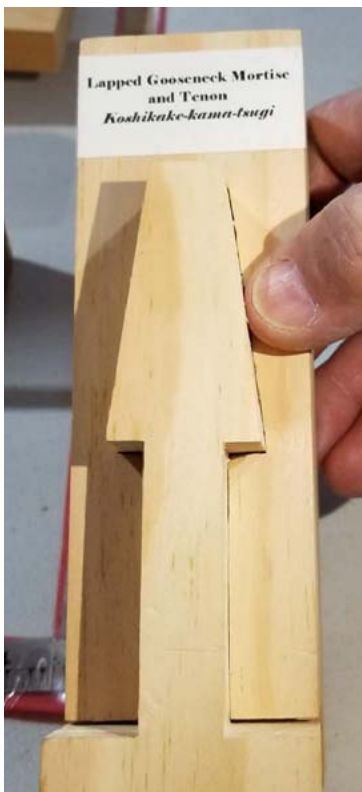
Lapped gooseneck mortise and tenon
