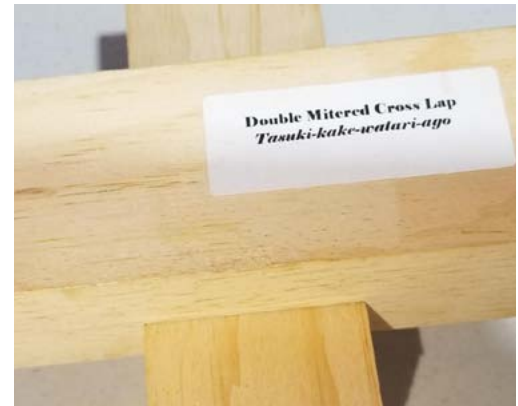
Double mitered cross lap
