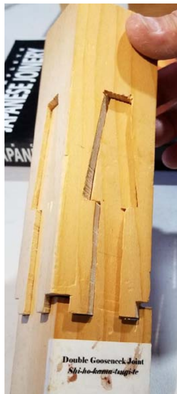
Double gooseneck joint
