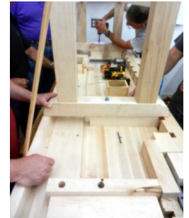
Assembling the 'H' frame legs
