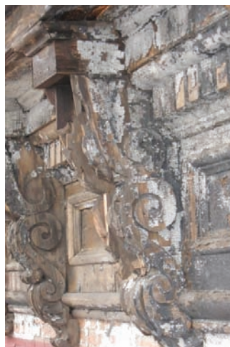
Original corbel on house, showing deterioration and missing parts.
