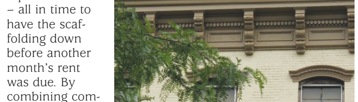
(FinishedRestoration.jpg) – Finished restoration, showing new corbels installed and painted.
